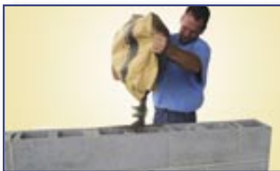
Loose fill is hard to handle and blows away easily in the breeze.
