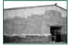
Figure 7: Effects of UV exposure. Lighter SPF was applied several days after the darker SPF.
