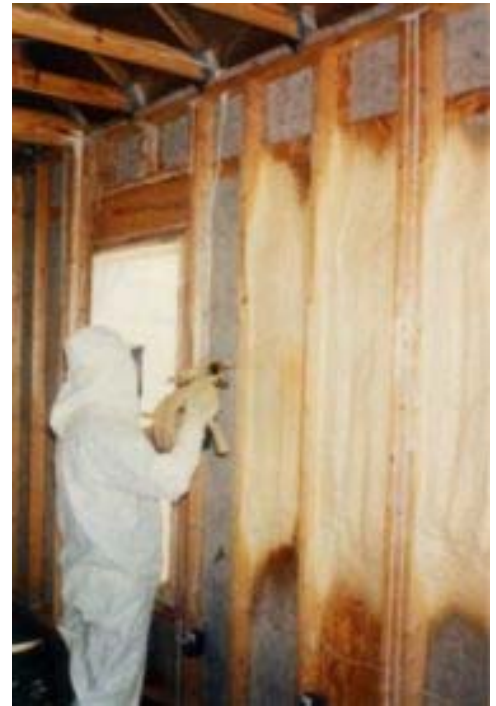
Application of NCFI 2020 PLUS to stud wall cavity.
